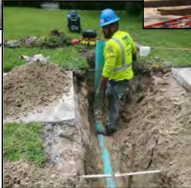
Installing sewer lateral
