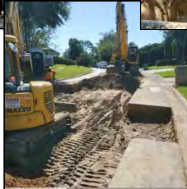
Installing roadway base
