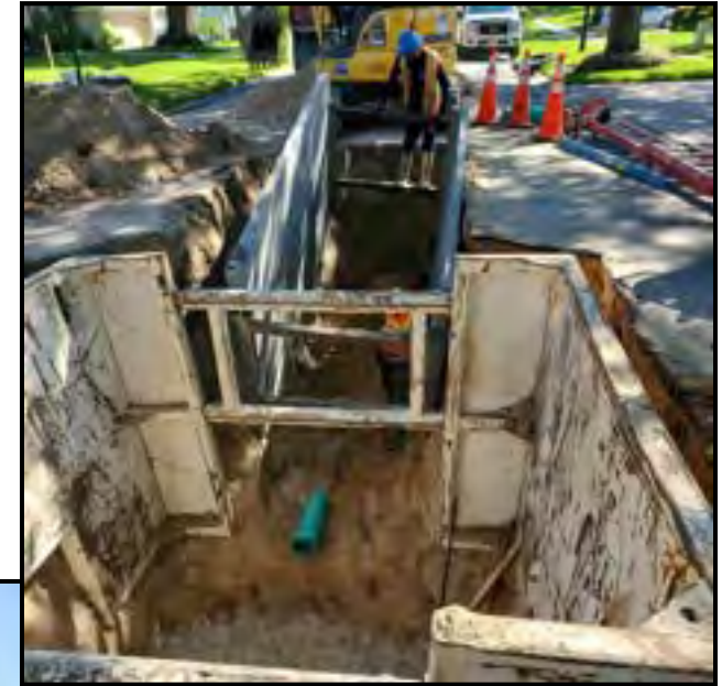
Installing gravity main
