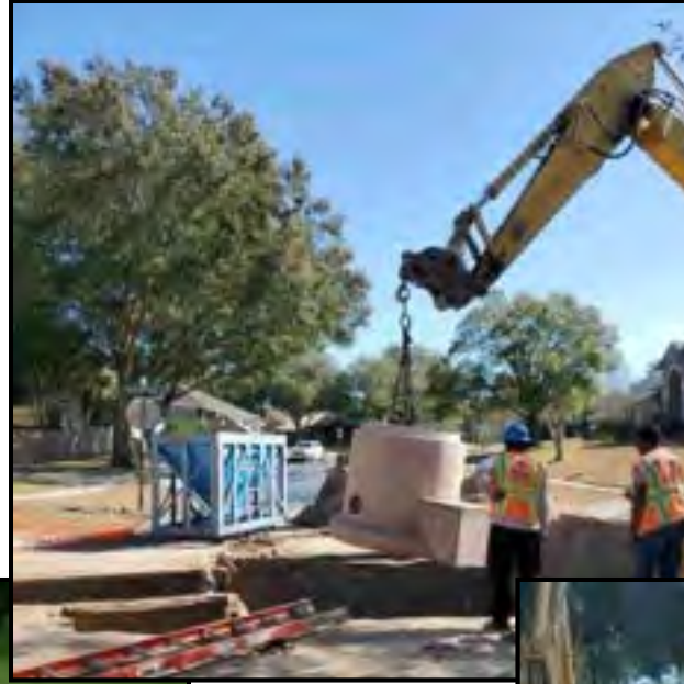
Installing manhole
