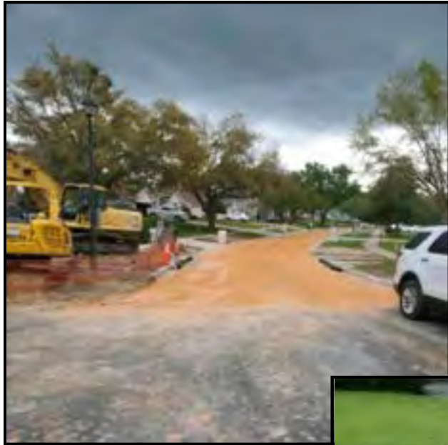
Installing roadway stabilization
